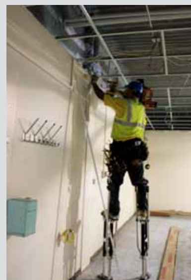
The asbestos abatement underway in Jones Physical Science Center
